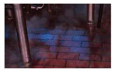
Concrete areas were first given a liberal coat of primer (PENNPRIME 101) which serves as the bonding agent for the glass-reinforced, 1/4 inch asphalt membrane. Then the membrane itself-a hot-melt, unfilled oxidized asphalt-was applied in several thin layers to a thickness of 1/4 inch and reinforced with a single-ply of open mesh woven glass cloth saturated with the same asphaltic compound.
